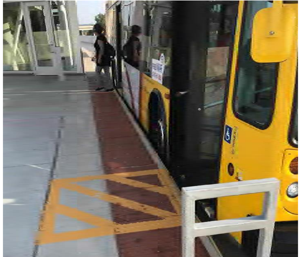
Level Boarding Platform Red Line BRT, Apple Valley, MN
