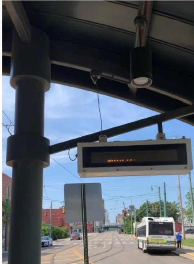
William Hudson Transit Center Station Overhead LED Variable Message Signs
