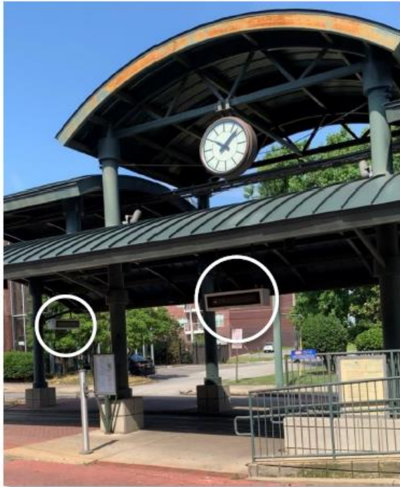
William Hudson Transit Center Trolley Station Overhead LED Variable Message Signs
